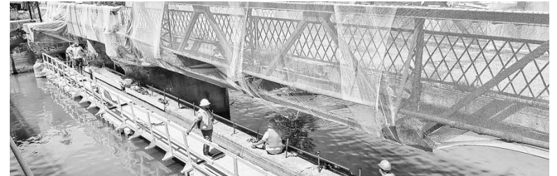
Repairs to Misner Dam were started earlier this summer.
